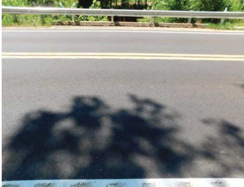
VIEW ACROSS TOP OF DECK
